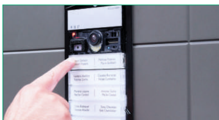
10. PRESS the button to which the address selected in the previous step will be assigned. An acoustic signal sounds to confirm that the address has been correctly assigned. By SELECTING the other buttons in succession, they automatically acquire the call address with the next code
