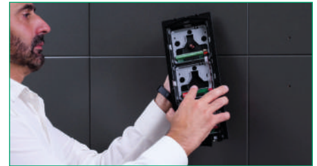
4. POSITION the surface-mounted entrance panel, guide the power supply wires through the appropriate slot and fasten it using the two screws at the top and bottom
